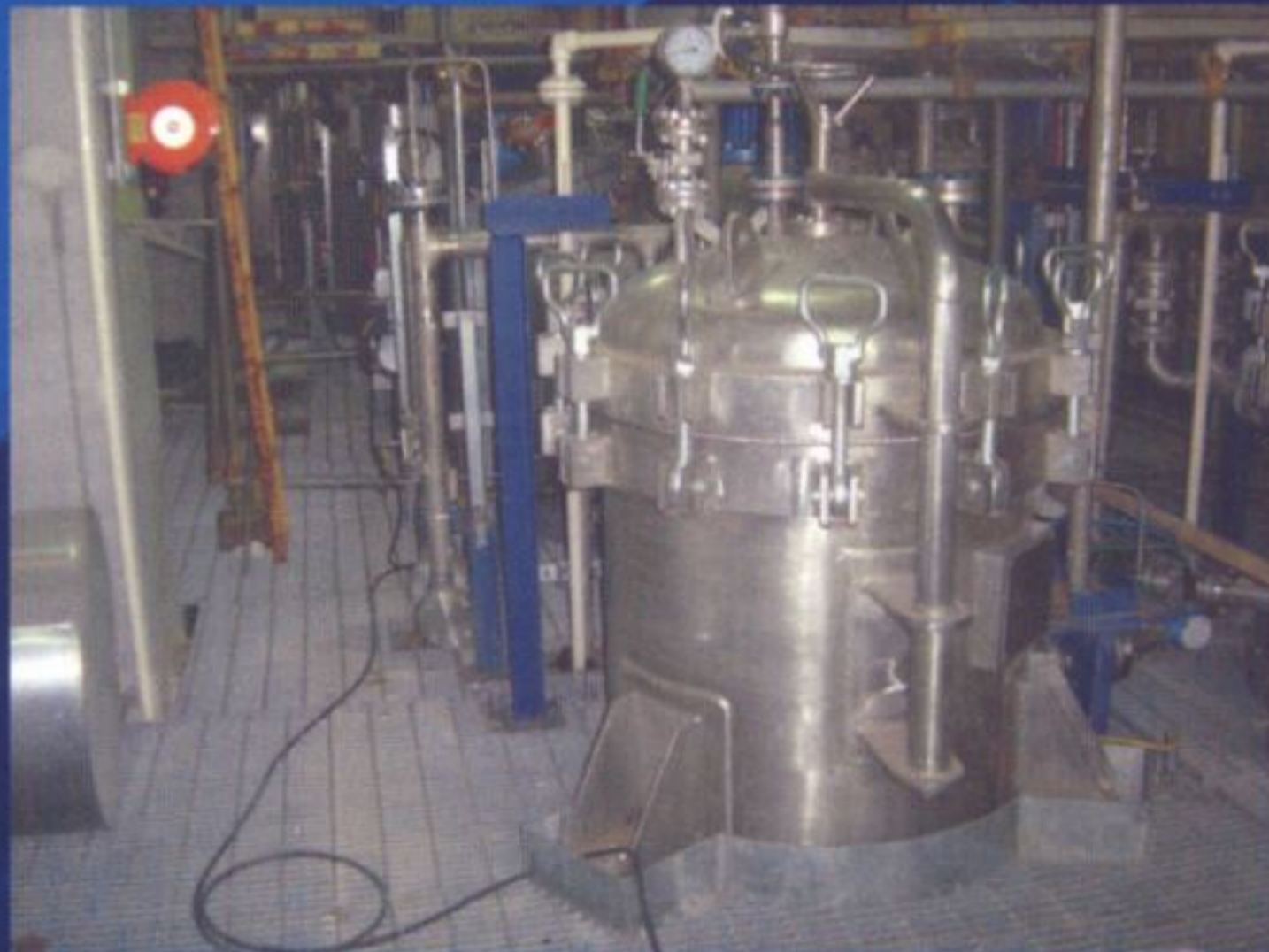
• Installation of Sharplex Pulsejet Candle Filter at Ciba Speciality, Singapore
